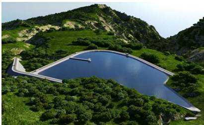
Upper reservoir, Barragem do Pico da Urze—1 000 000 m 3 (photo courtesy of EEM)
