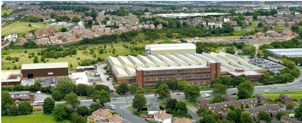
AH product manufacturing and testing plant in Leeds, UK
