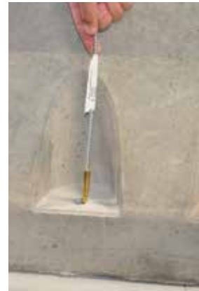
Figure 5d: Brush out borehole
