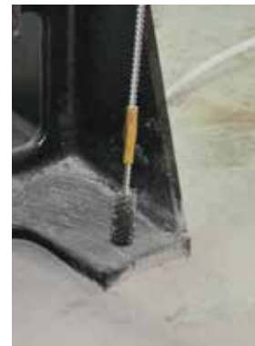
Figure 8d: Clean bore holes
