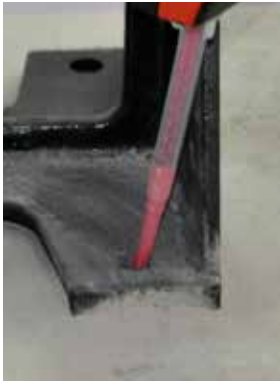
Figure 9a: Fill with composite mortar
