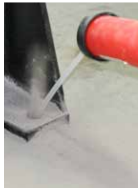
Figure 8c: Set bore holes
