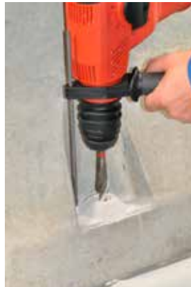
Figure 5b: Drill the fixing holes
