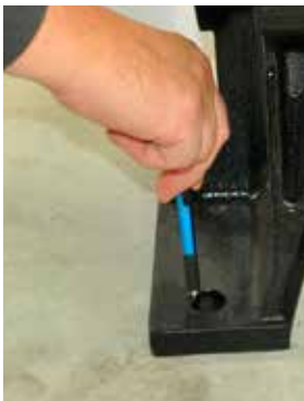
Figure 8a: Mark bore holes
