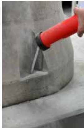
Figure 5c: Blow out the borehole
