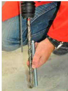
Figure 8b: Set bore holes
