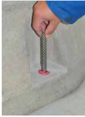
Figure 6b: Insert the reinforcement
