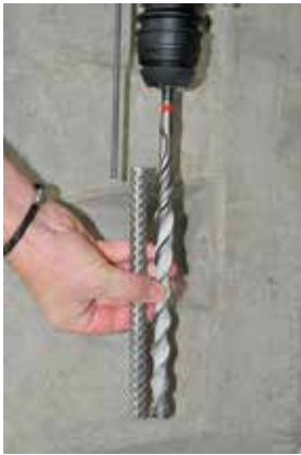
Figure 5a: Set the drill depth
