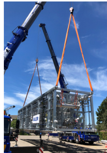
Skid mounted module: from 3-D layout to final plant
